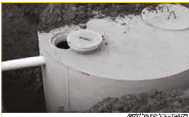
Figure 51: Pipe connection to precast septic tank
