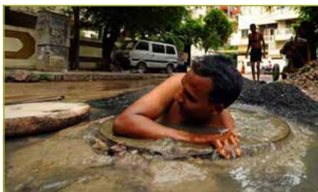
Figure 69: A sewerage worker clears a choked drain
