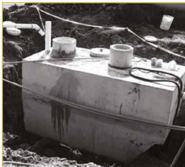
Figure 53: Installation of precast septic tank
